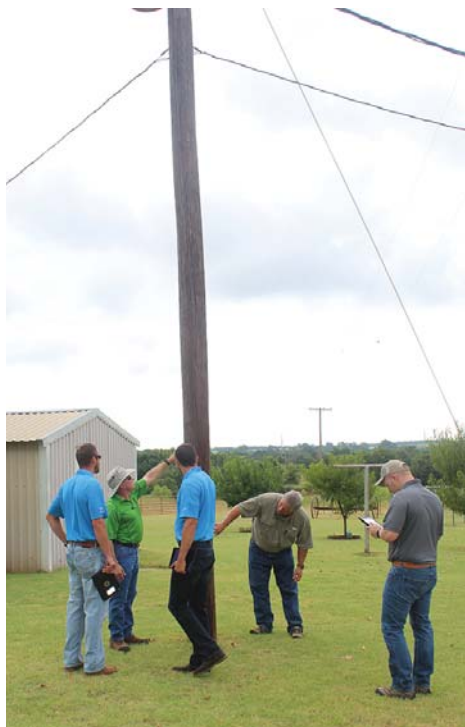
REC employees have begun working on site locations for the new radio frequency advanced metering infrastructure.
