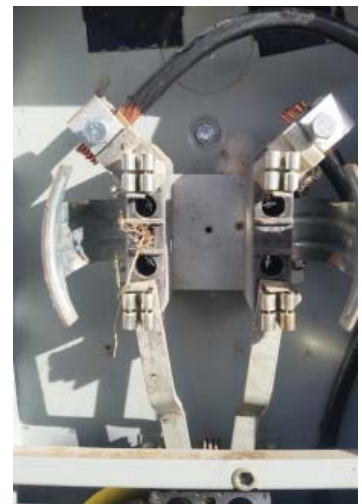
During the process of Chapman Metering changing the meters, they are also doing preventative maintenance. While changing the meters, they take pictures of the old meter (left), the new meter (middle) and the sockets (right) and conduct a hot socket test.
